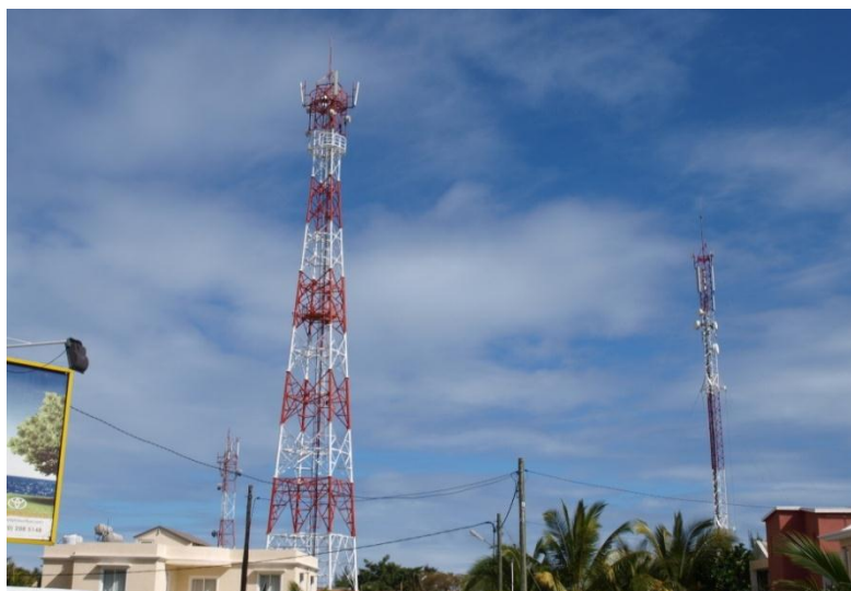
Figure 1: Standalone lattice steel structure
